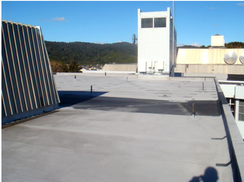
Picture – an example of Greymouth Hospitals flat roof.
