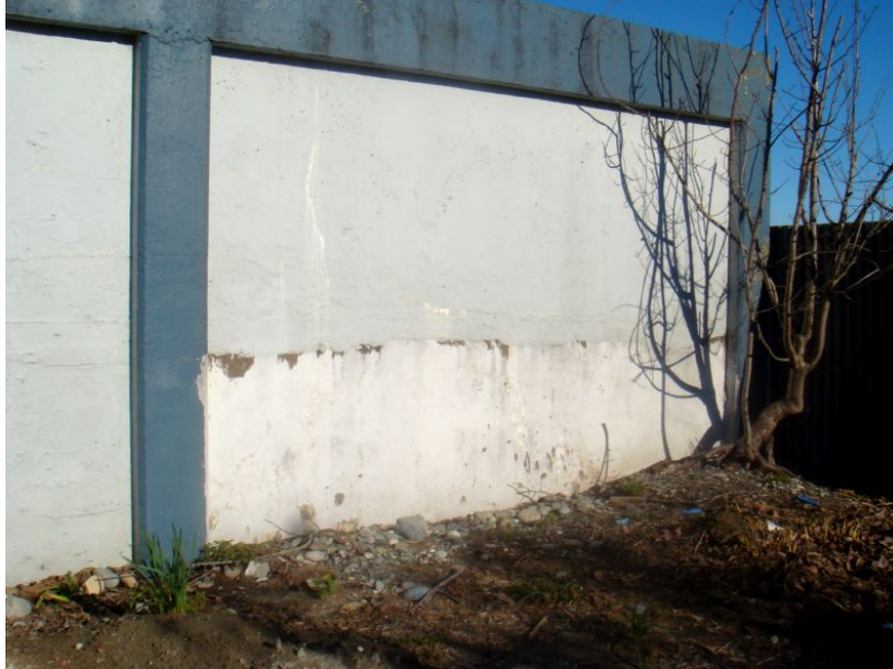
Picture – visible cracks in the water tank which acts as Greymouth Hospital's emergency water supply.
